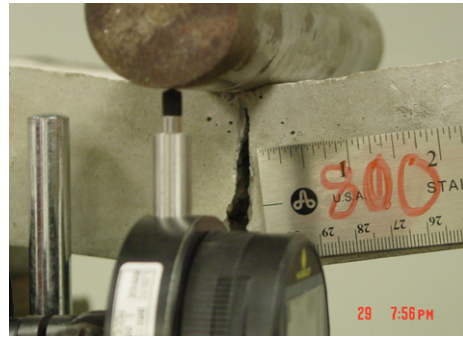
Figure 5. During loading: the crack can be obviously seen.
